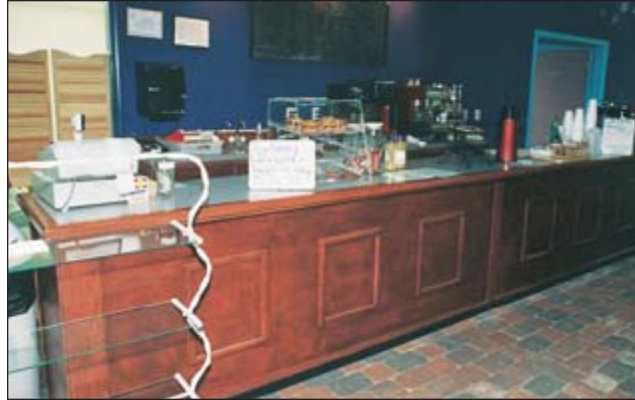
This food service bar is part of the woodwork Johnson has done for a Lynchburg, Va., bookstore. Other work in the store includes fixtures, displays, checkout counters and more than 160 bookcases.
